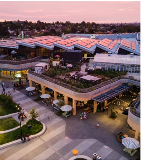
Burwood Brickworks Melbourne
