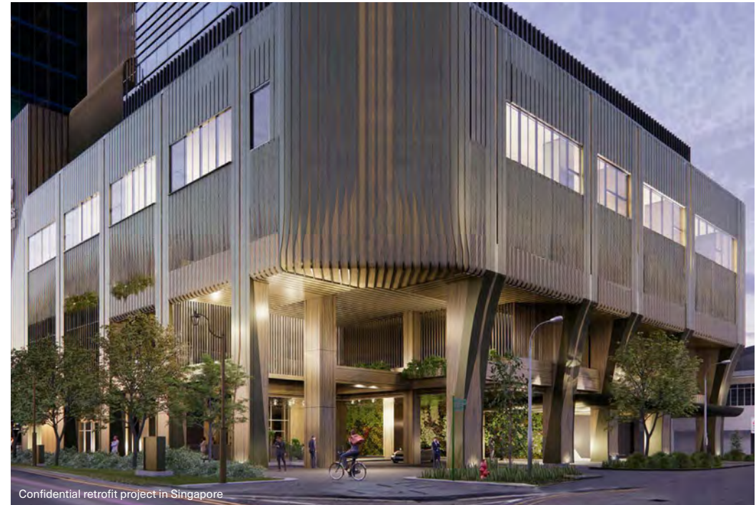
Confidential retrofit project in Singapore
