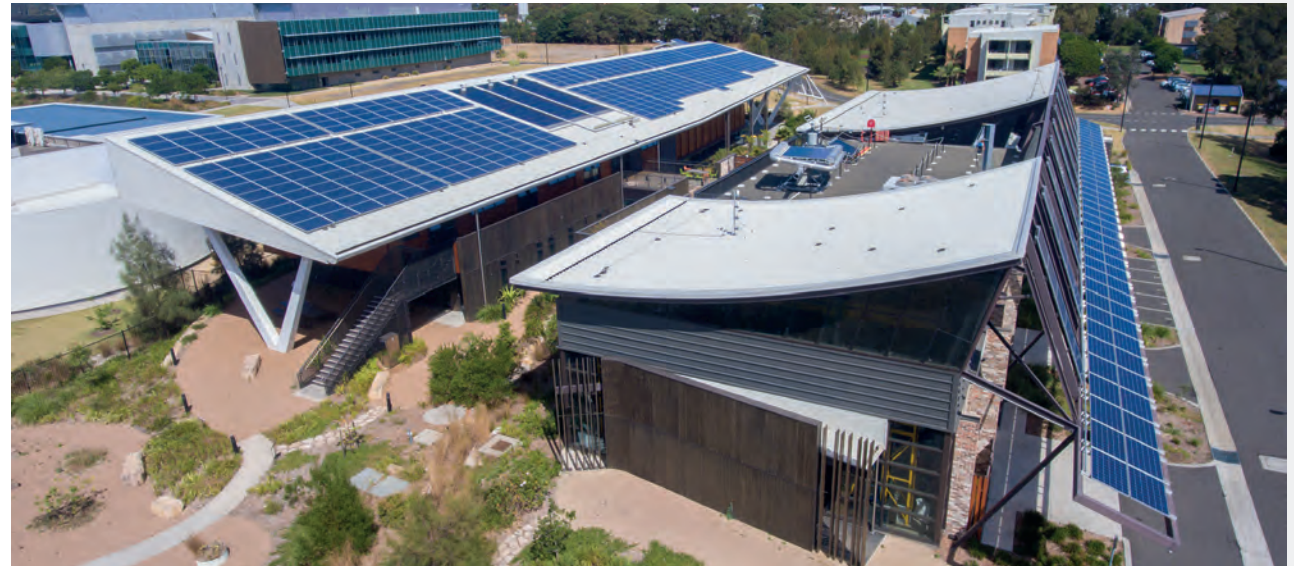
Sustainable Buildings Research Centre, University of Wollongong © Matt Estherby
