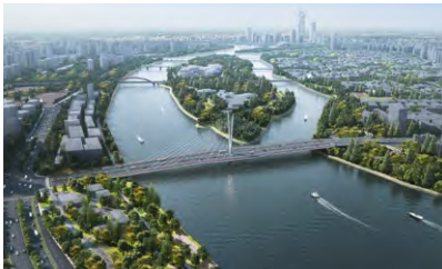
2023 International Architecture and Design Awards Arches, Bridges, Viaducts, and Gateways Architecture Concept Jinhua Hepan Bridge - Bronze
