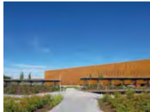
Northern Sweden DC2 Luleå, Sweden
